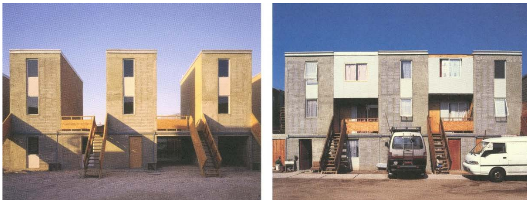
Figure 6.1. Quinta Monroy dwellings, before and after homeowner extensions (Aravena 2010, 88).
