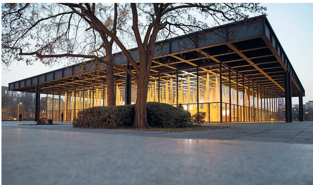
Figure 3.1. Neue Nationalgalerie Entrance Pavilion (Carsten, 2014).
